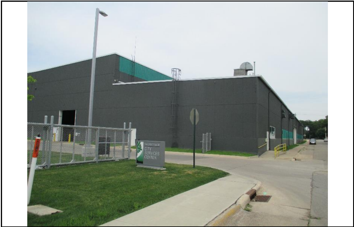
Photo 1: View of Building 16 roof access, looking north.
