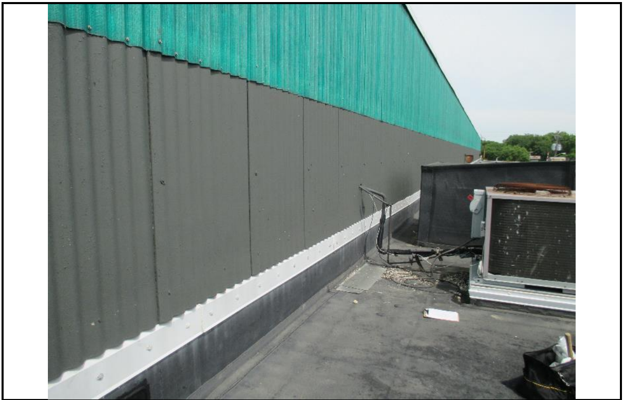
Photo 10: Picture of the asbestos cement board siding on the building.
