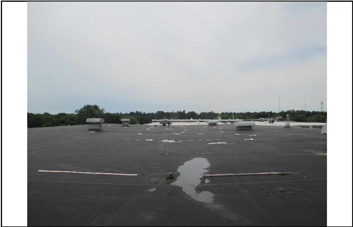
Photo 5: View of upper roof looking north.
