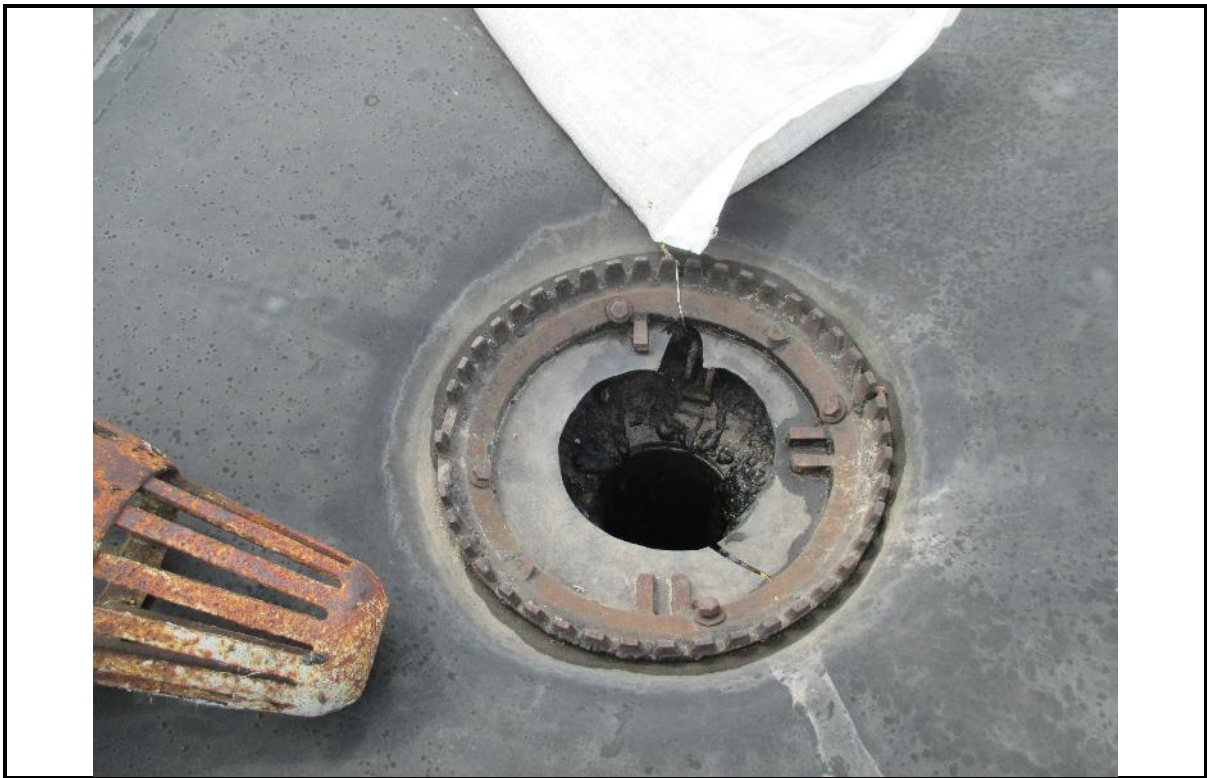
Photo 8: Picture showing the bituminous coating in the upper roof drains.
