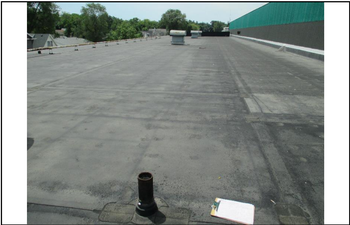
Photo 2: Picture of cast vent penetration with ACM flashing on lower roof, looking south.
